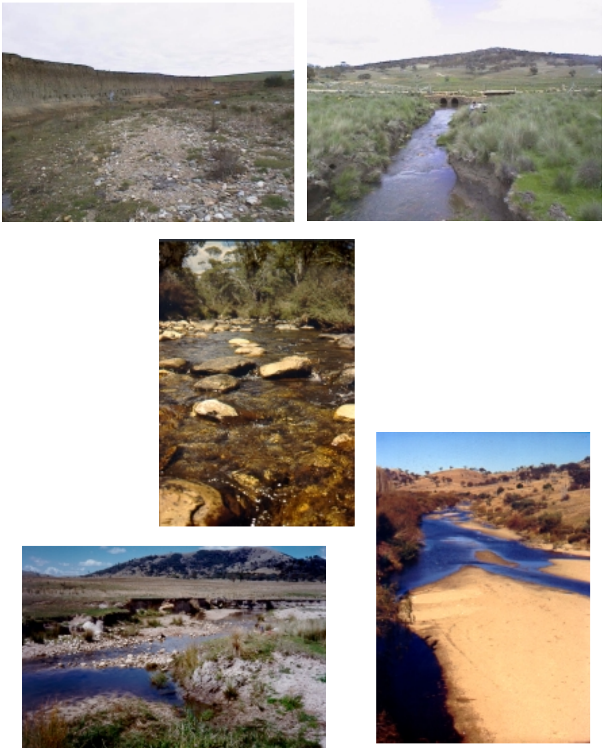
Figure 5.21 Examples of bed stability. Severe erosion (top left), moderate erosion (top right), bed stable (centre), moderate deposition (bottom left) and severe deposition (bottom right).
